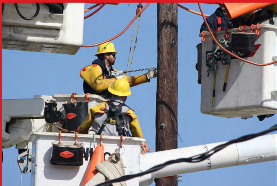
Lineman drills into a distribution pole, 2022. Garland Power & Light Collection
