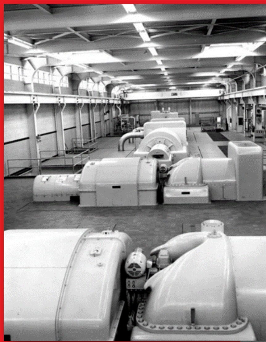
Turbine generators inside Newman Power Plant, 1967. Garland Landmark Museum Collection
