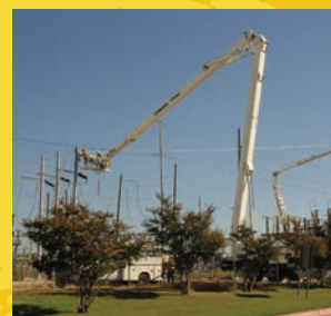
Fiber optic shield wire upgrade
