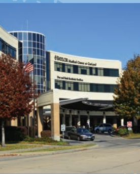
Window tinting for energy efficiency
