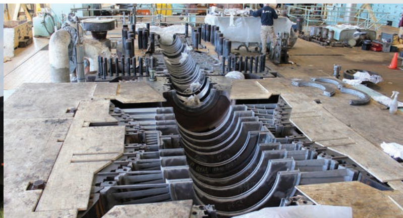
Olinger Unit #3 outage
