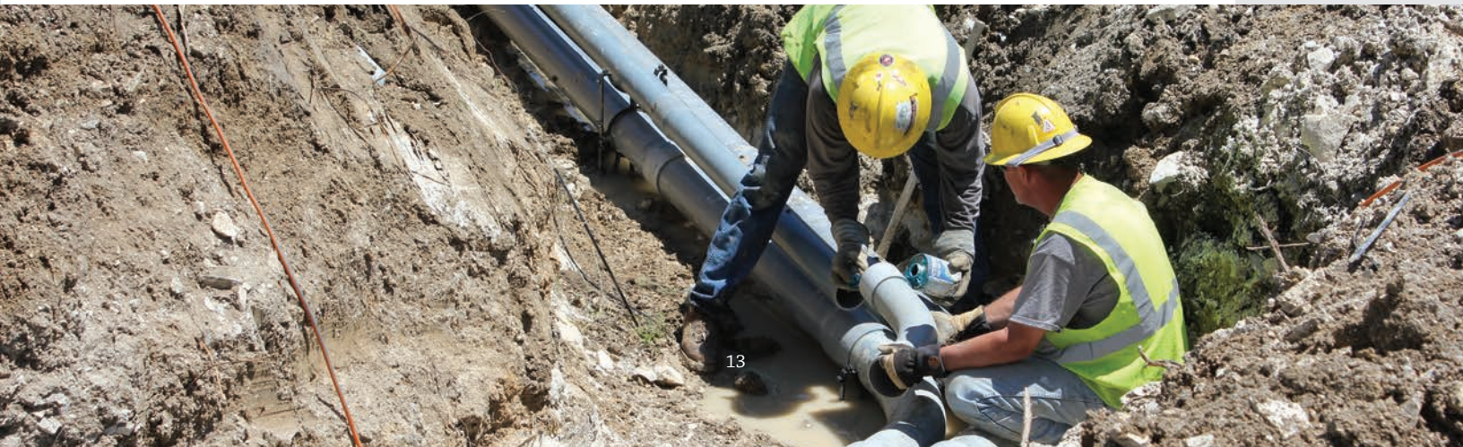
600-amp feeder loop in north Garland
