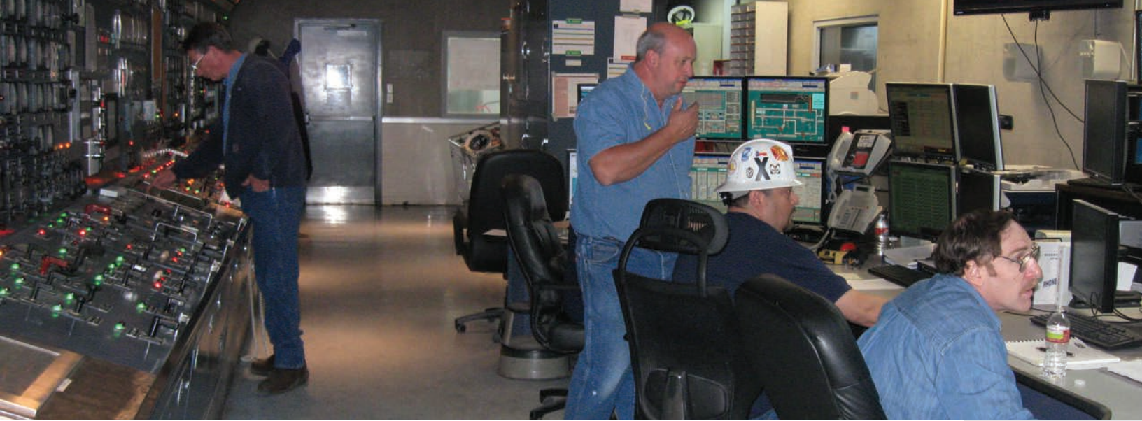
Olinger control room
