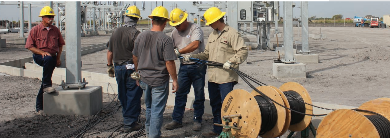
Transmission switchyard construction near Nevada, Texas
