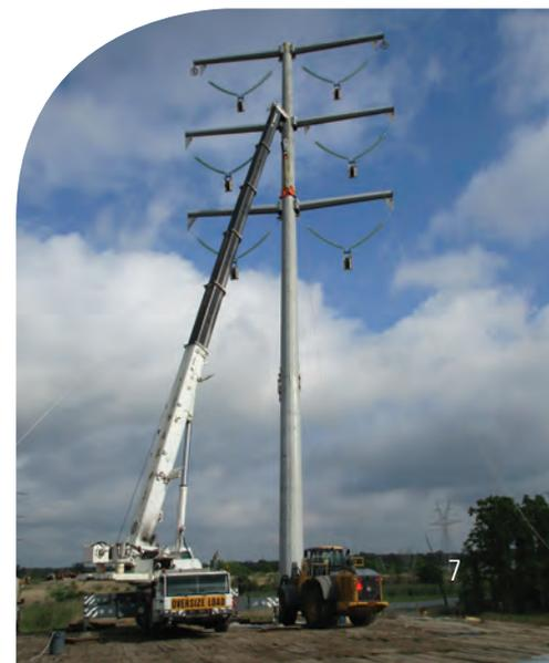
In West Texas, GP&L conducted thorough inspection and maintenance of the utility's 75 miles of transmission line in the Competitive Renewable Energy Zone. Maintenance activities included the replacement of some davit arms and installation of vibration dampers.
